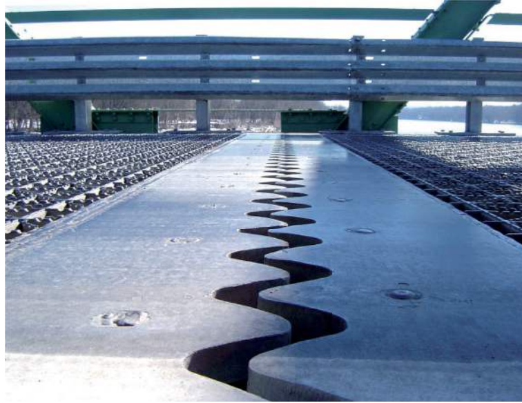
Figure 6: Expansion joint on a bridge
